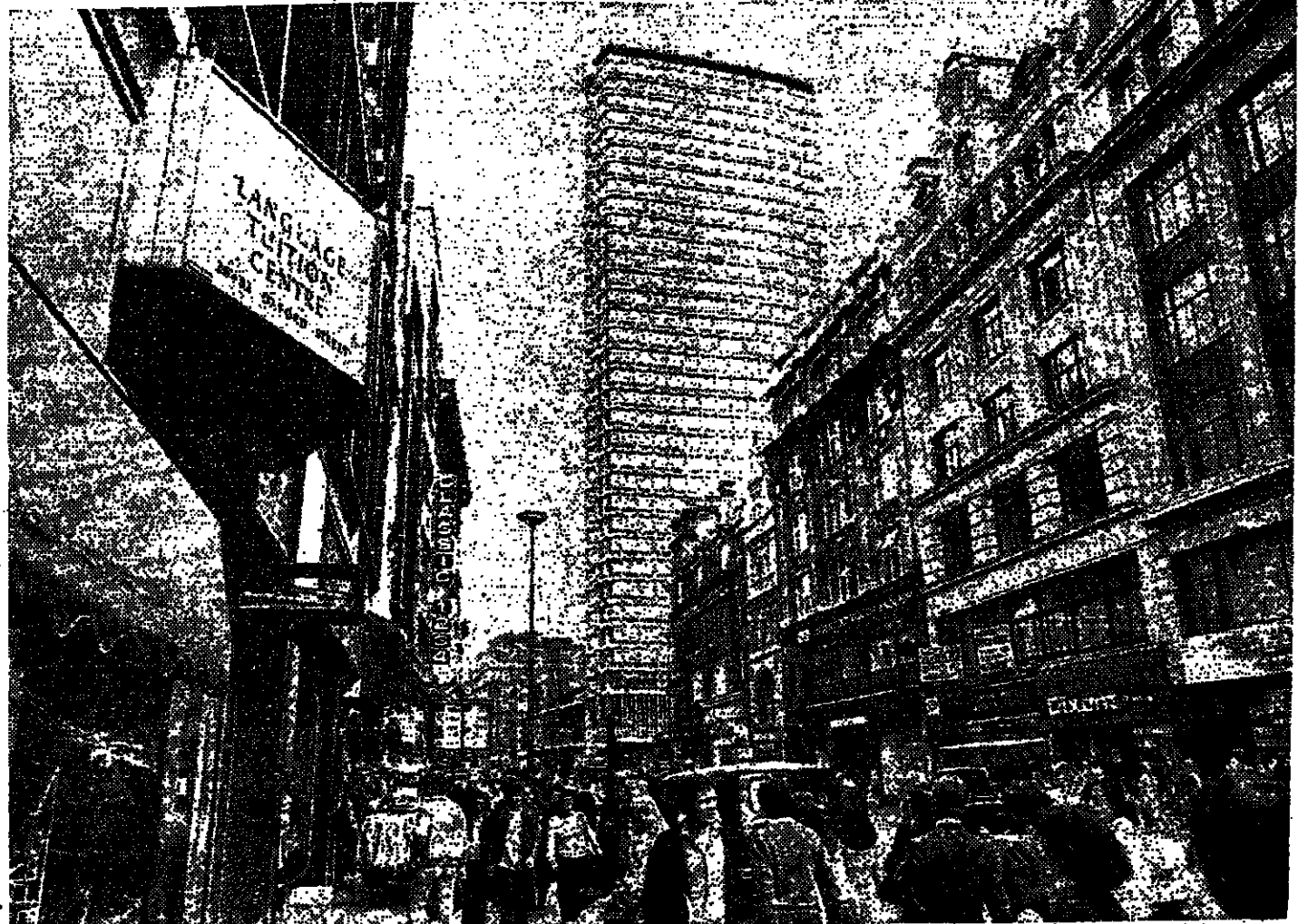
The CBI has leased 103,000 sq ft of Oldham Estates' Centre Point (seen here from Oxford Street) at a rental of just over £7-a sq ft on a 45-year lease
